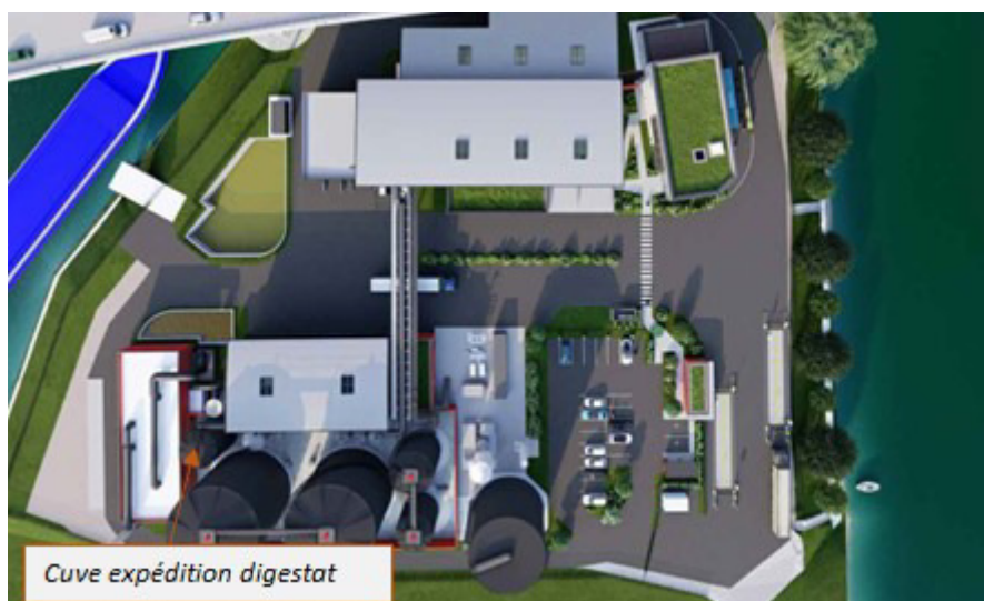
Figure 42. Cuve de stockage tampon digestat
